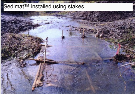
Disturbed sediment entering Sedimat™
