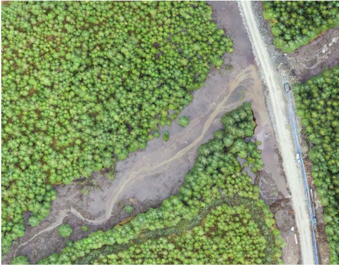
Figure 2.2 Aerial image of water and peat impoundment area upstream of Wall 1 showing large volumes of impounded peat and clearly identifiable channel for water reaching Wall 1
