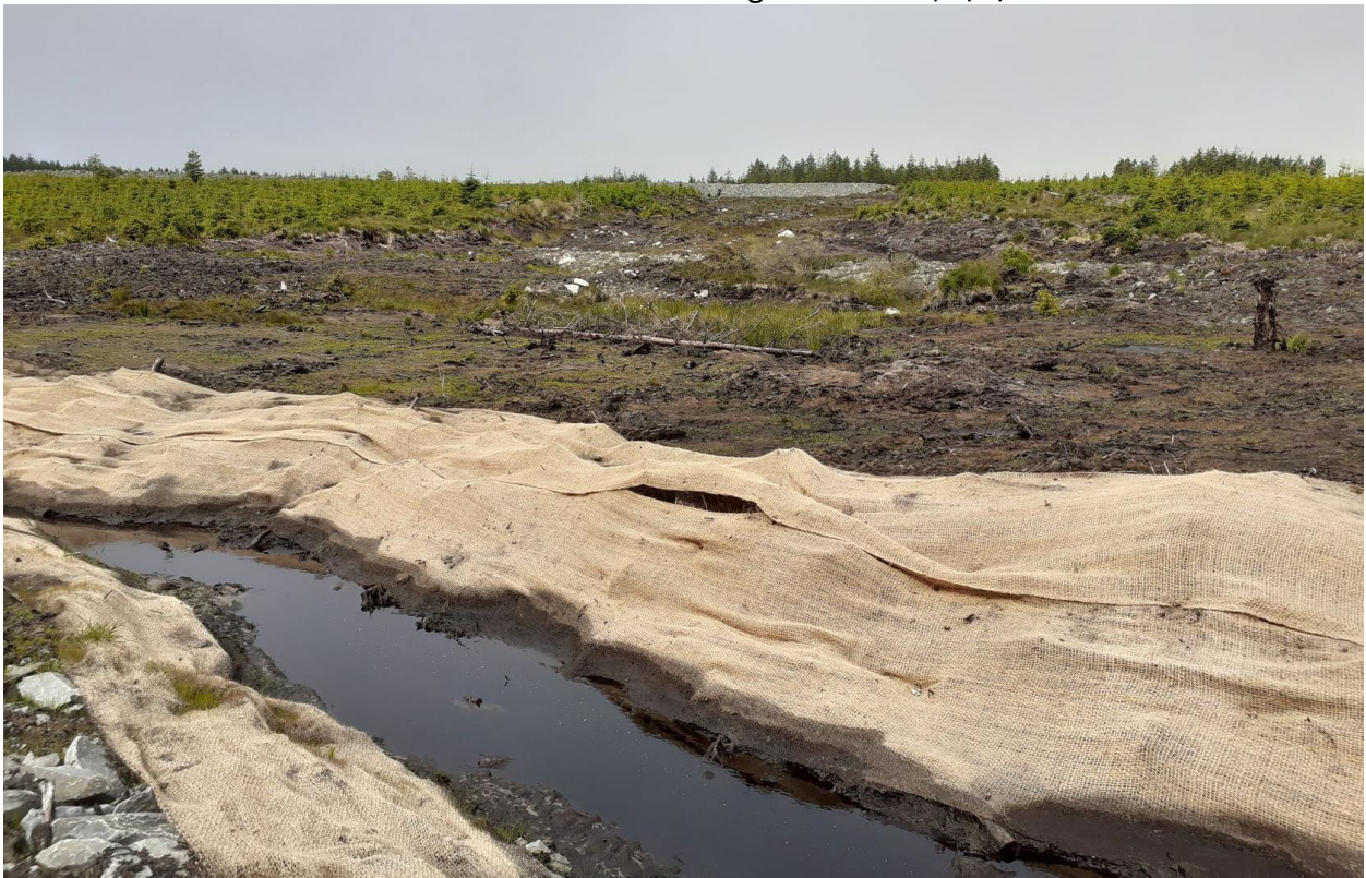
Photo 5 - Sruhingarve stream, looking up towards Wall 3, 8/7/22
