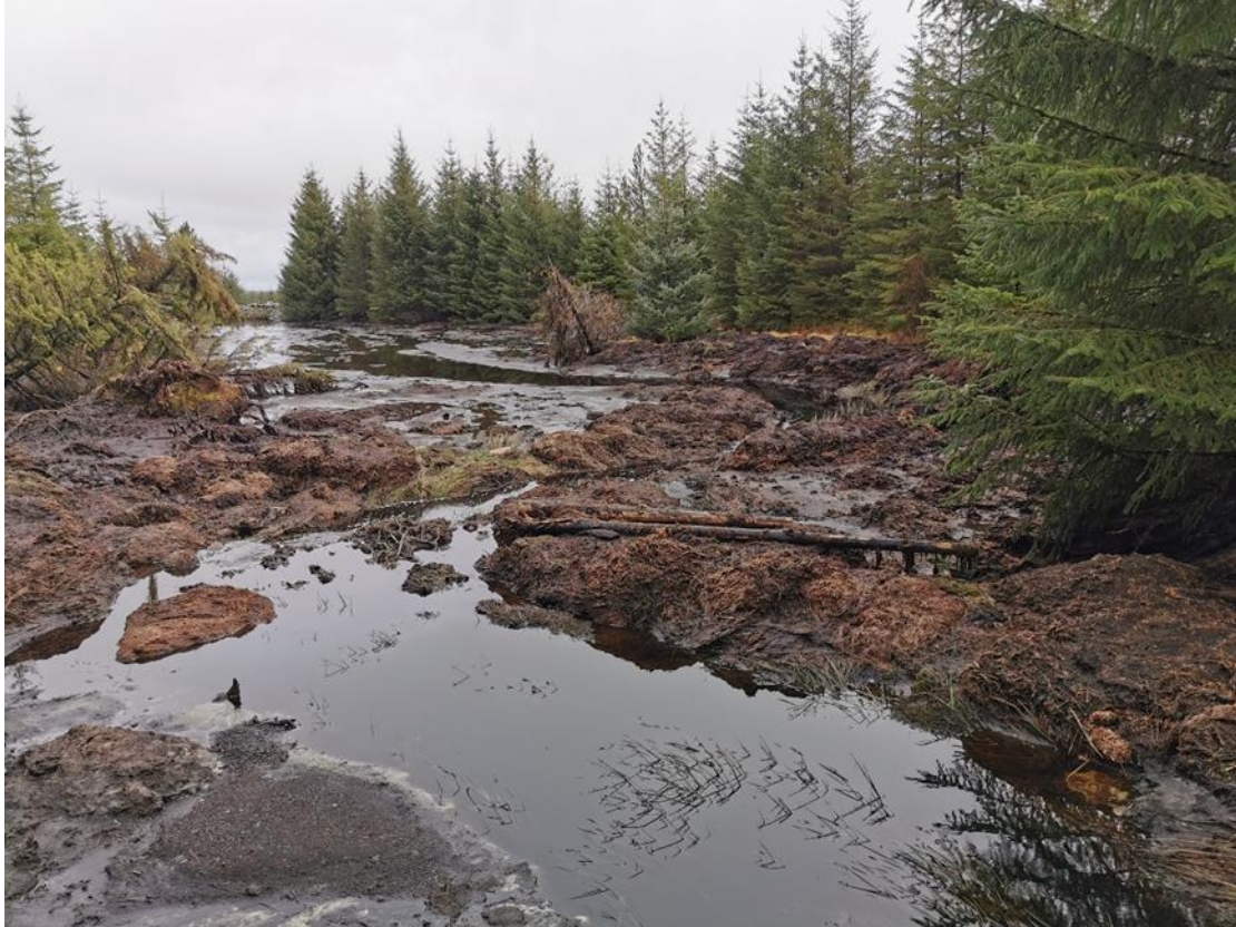
Plate 2.3 View of impounded area prior to commencement of sediment removal works, facing downstream
