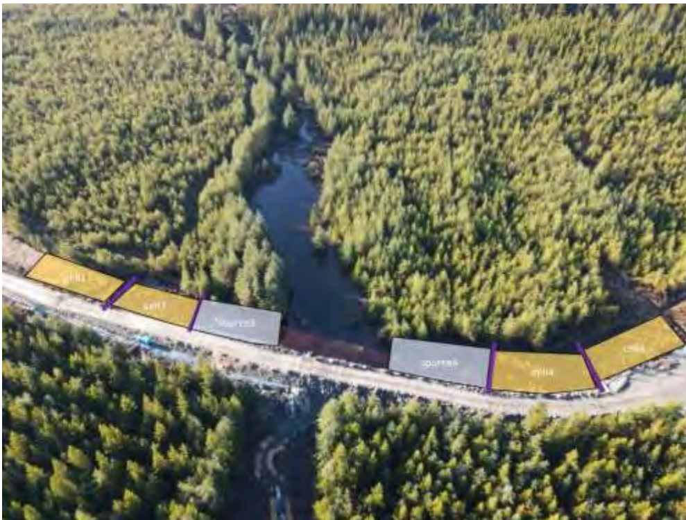
Figure 5.15 Creation of intermediate drying cells
