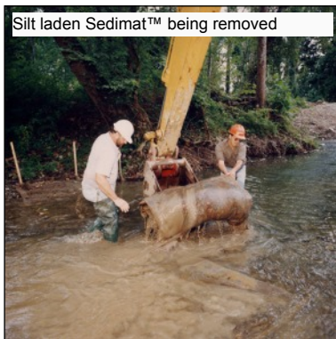
Trapped silt in Sedimat™
