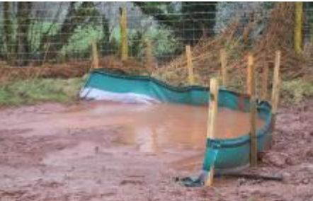
Hy-Tex Terrastop silt fence in use on National Grid's Felindre to Brecon gas pipeline project
