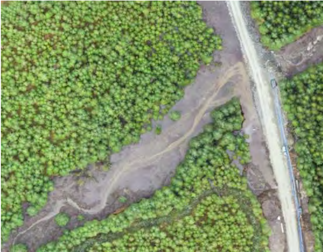
Figure 2.3 Aerial image of water and peat impoundment area upstream of Wall 1 showing large volumes of impounded peat and clearly identifiable channel for water reaching Wall 1
