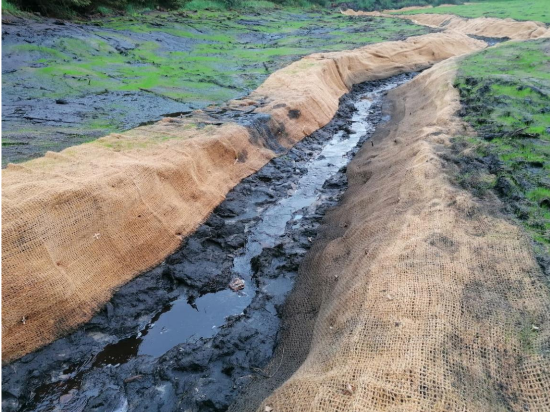
Plate 2.6 View of coir matting installed on re-established stream channel, facing upstream
