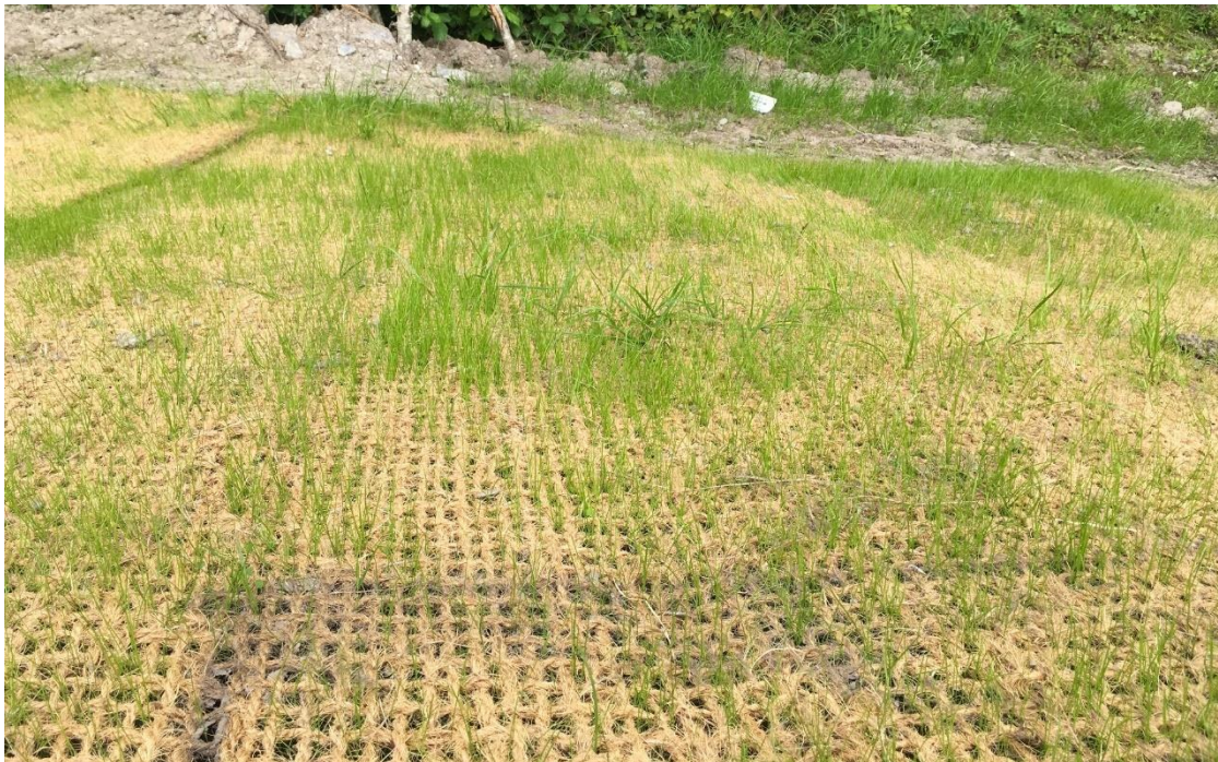
Figure 5.10 Grass growing up through CoriMesh on previously bare soil surface.
