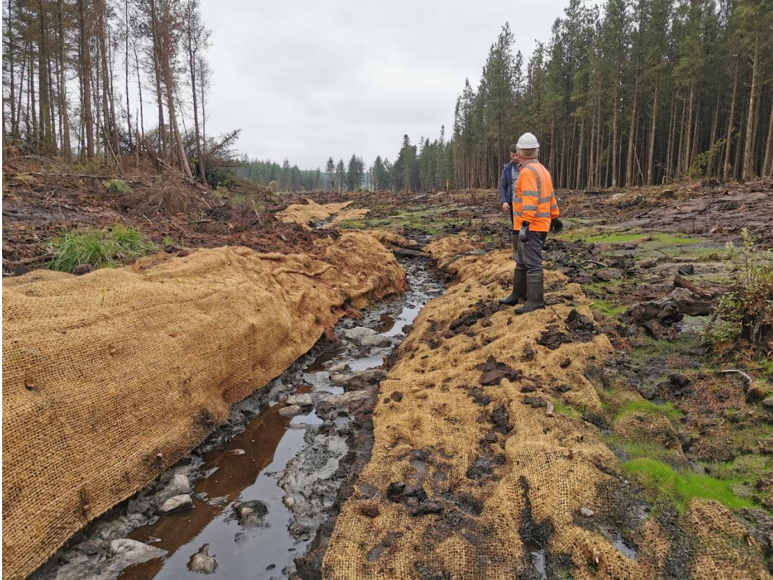
Plate 2.2 View of Reach 2 (Upper) following removal of dangerous trees, facing upstream.
