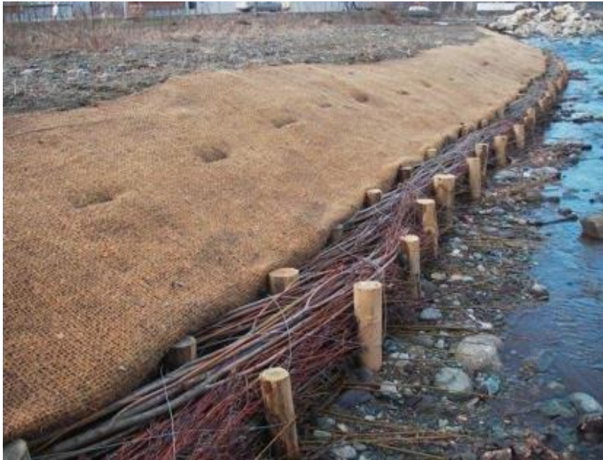
Plate 3.4 Live willow fascine installed at toe of bank.
