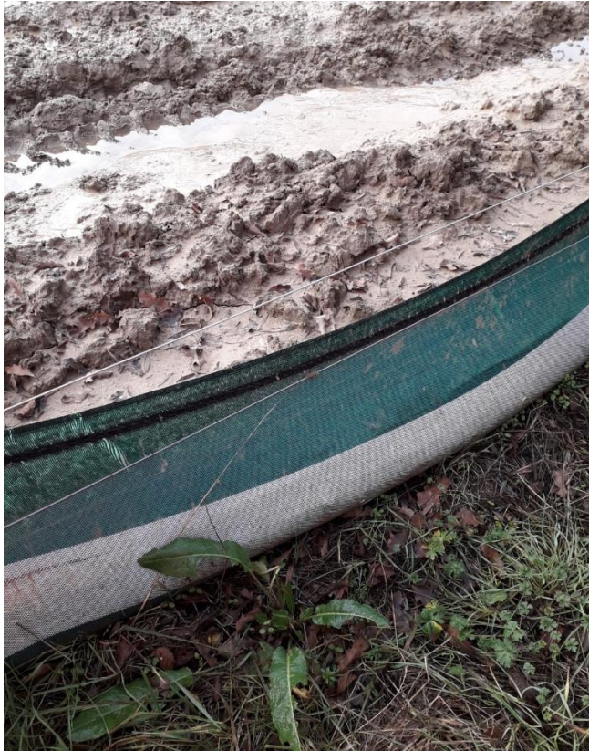
Figure 5.7 Terrastop silt fence properly buried into ground surface acting as effective silt barrier
