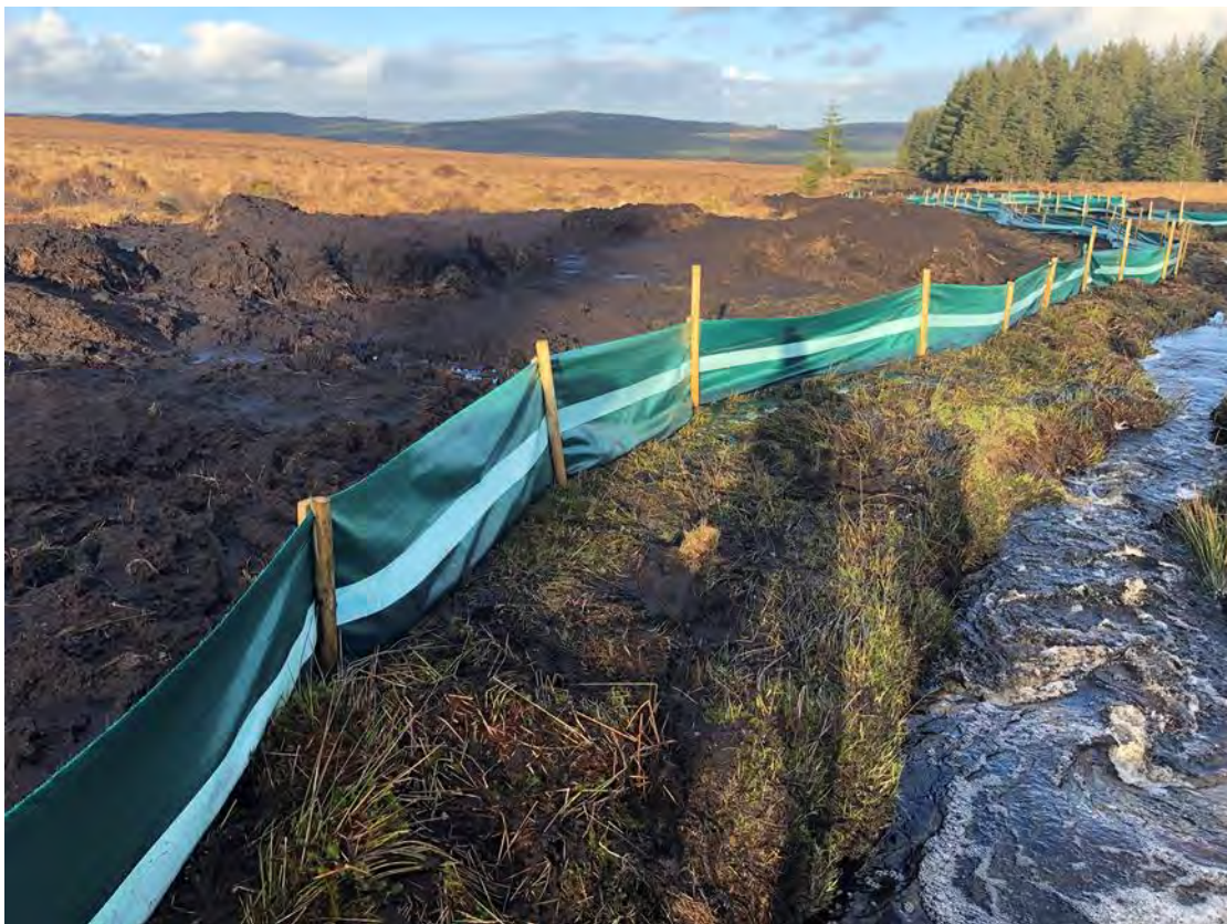
Figure 5.10 Silt fence Installed on Reach 4
