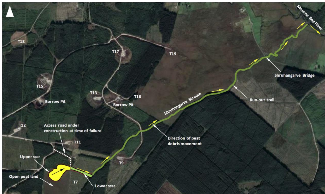
Figure 1 Extent of peat failure of 12 November 2020
